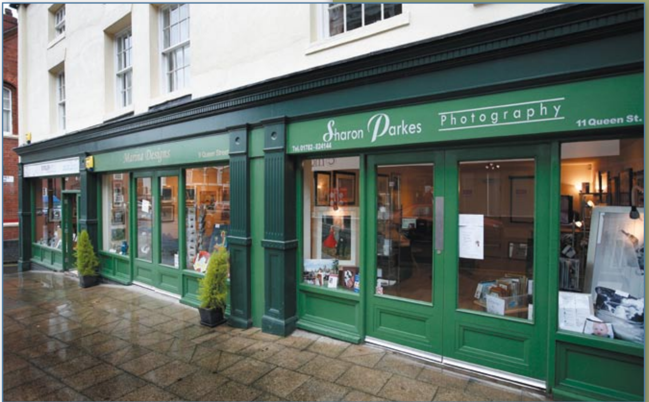
The first phase live/work units are above creative retail spaces on the ground floor
