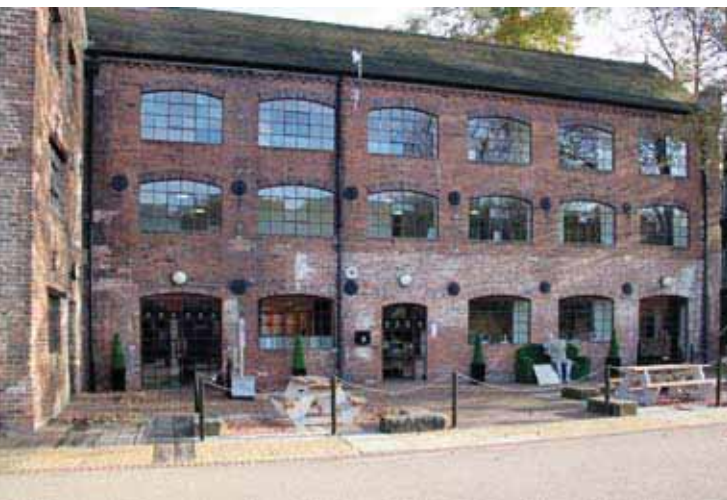
The Enterprise HQ building, originally a china factory, is owned by a museum trust and leased out as a workhub
